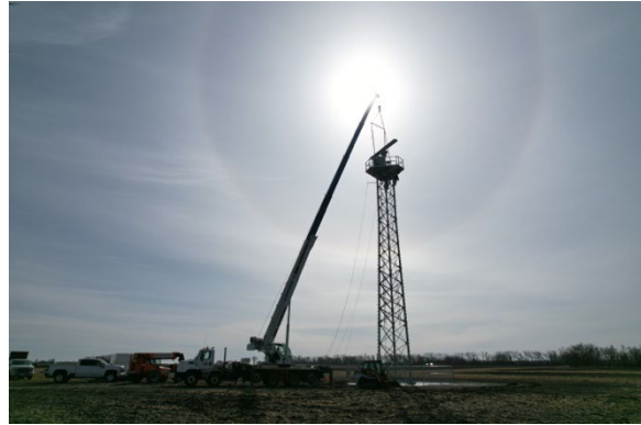
Figure 10: Full View of the Installation of a Terma Radar in ND as Part of the Vantis System
