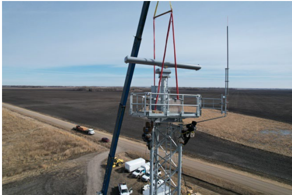
Figure 9: Installation of a Terma Radar in ND as Part of the Vantis System
